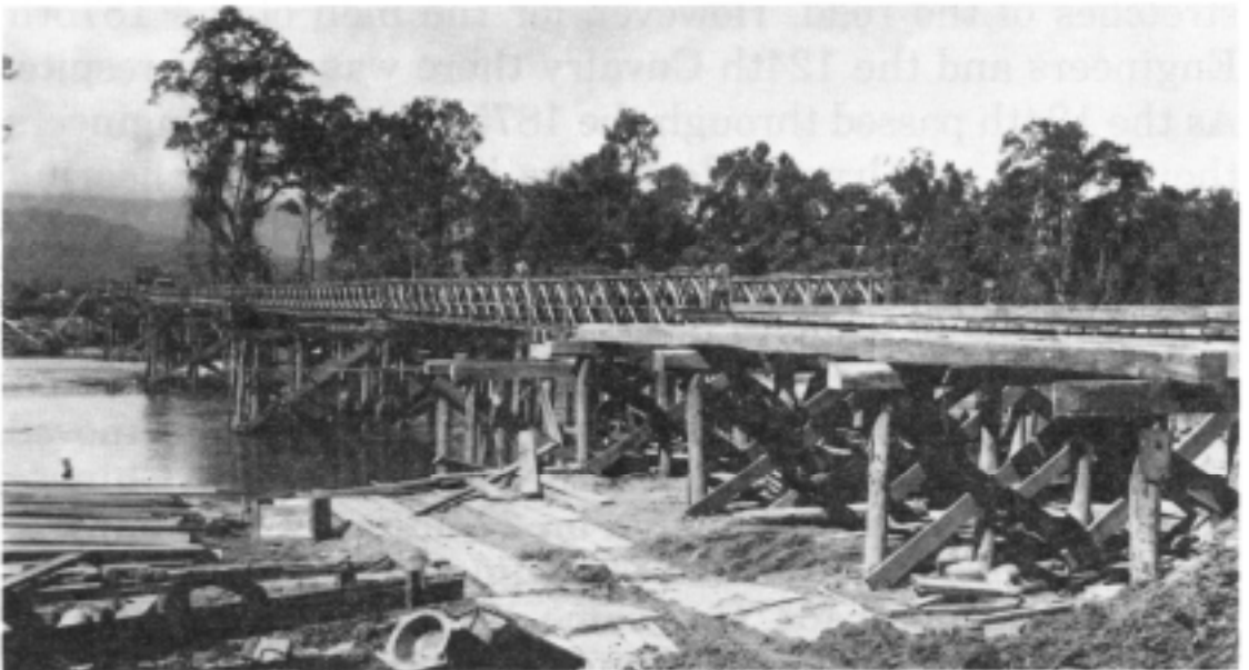
Construction of a Bailey bridge over the Mogaung River south of Warazup, Burma.
