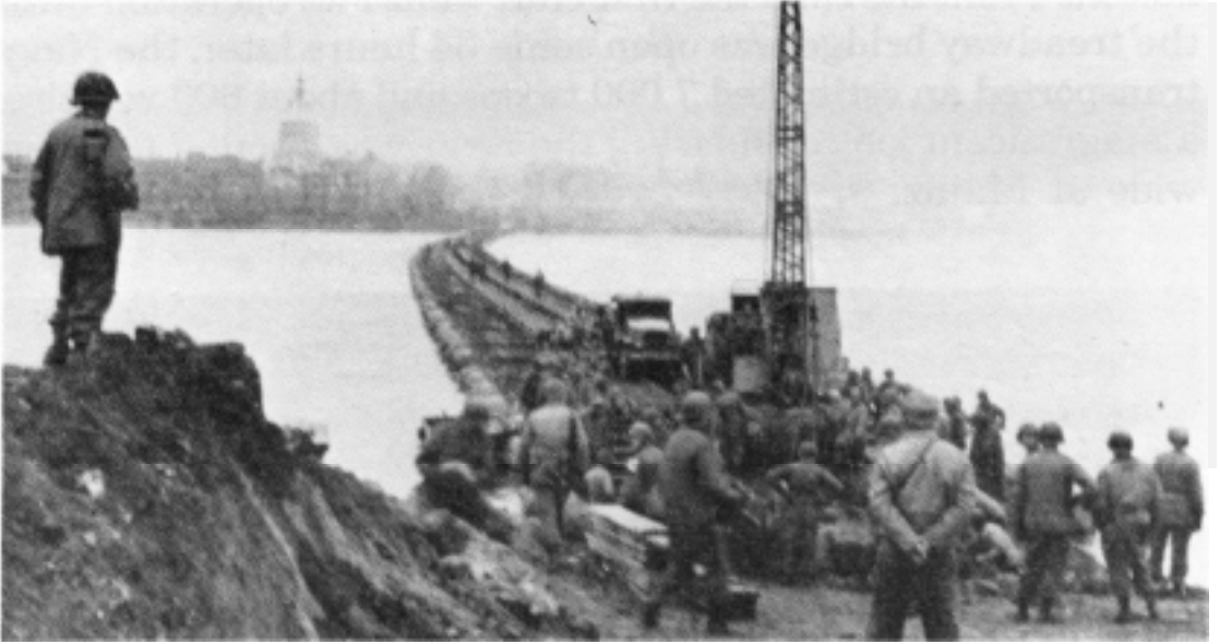
The 160th Engineer Combat Battalion built the longest tactical bridge across the Rhine at Mainz, Germany, 23 March 1945.
