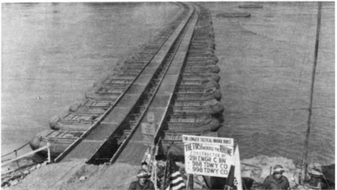
The first tactical bridge across the Rhine built by the 291st Engineer Combat Battalion and two treadway companies spans the Rhine River between Remagen and Erpel, German. PFC Vernon H. Bradberry and PFC Clinton E. Farmer form a color guard, 19 March 1945.
