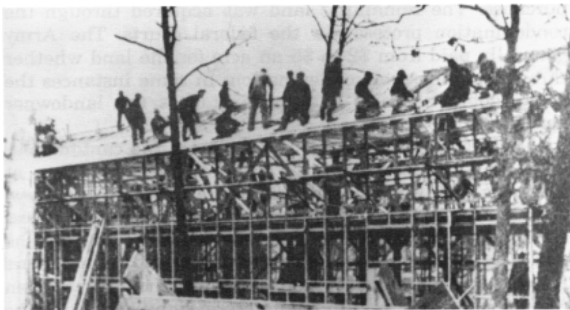
Construction of one of the 600 barracks built at Fort Leonard Wood, Missouri, 1941.
