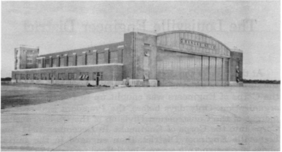
Completed hangar for Air Corps operations, Godman Field, Fort Knox, Kentucky, 6 October 1941.
