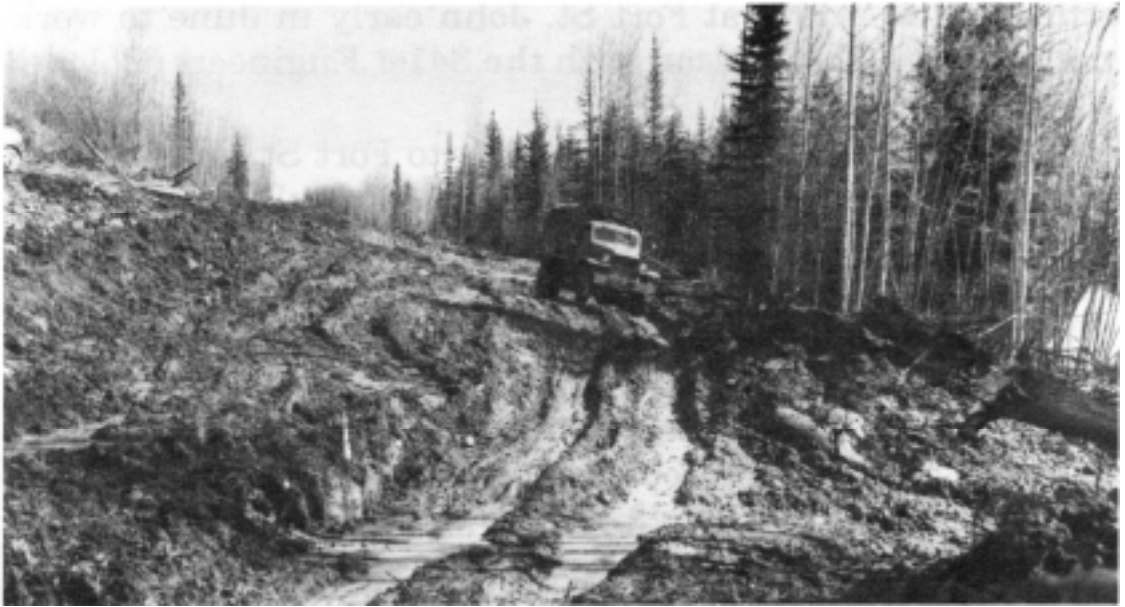
The 18th Engineers began working north from Whitehorse in late April 1942. The conditions on the cleared but ungraded and unfinished road hampered the movement of men, equipment, and supplies (National Archives)
