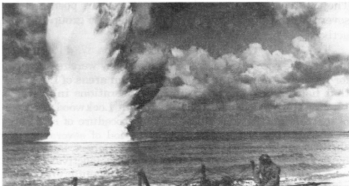
Company D, 373d Engineer General Service Regiment blows German concrete barges underwater. Staff Sergeant Thomas Atchison detonates the charge Le Havre, France, 1 October 1944.
