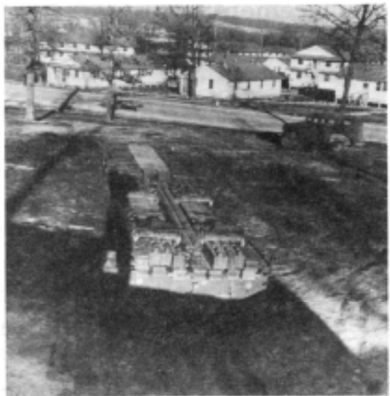
The 89th Engineers loaded portions of a 25-ton ponton bridge on a trailer, Fort Leonard Wood, Missouri, January 1942.
