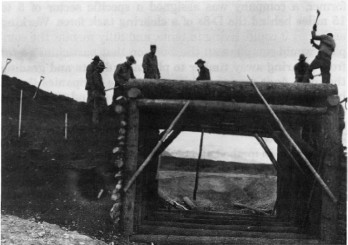
Timber box culverts were used in great numbers along the Alaska Highway. Timber was plentiful and used generously for every possible application.
