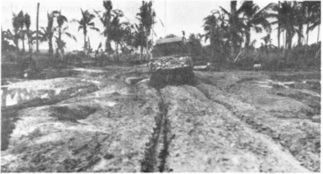
Poor drainage, heavy rains, and military traffic made maintenance a problem on Highway 1 going north from Burauen, Leyte Island, 5 December 1944.
