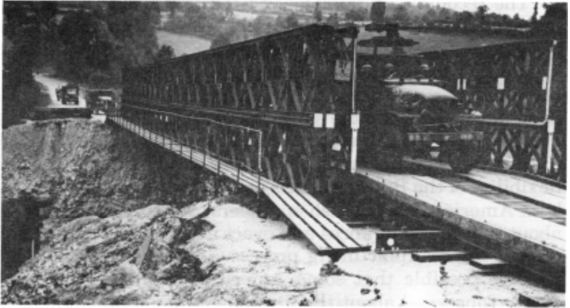
Traffic crossing a class 70 panelbridge with a pedestrian walk. (Engineer School Library)
