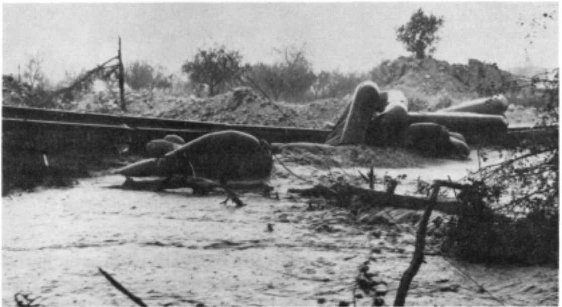
A wrecked ponton bridge washed out by flood waters on the northern Volturno River.
