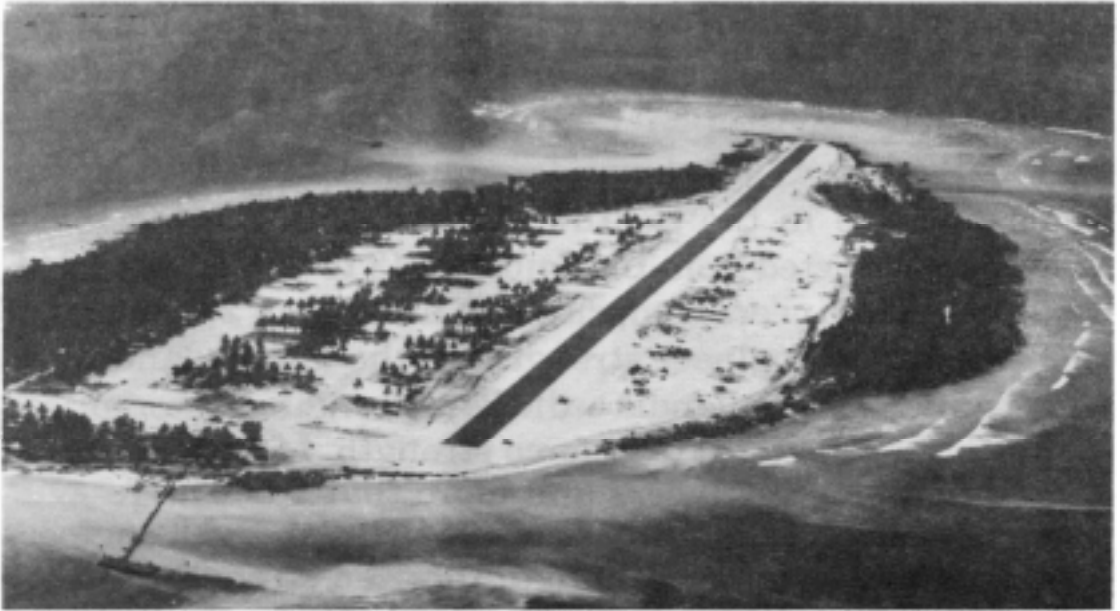
Aviation engineers construct an airfield stretching the entire length of Middelburg Island, September 1944.
