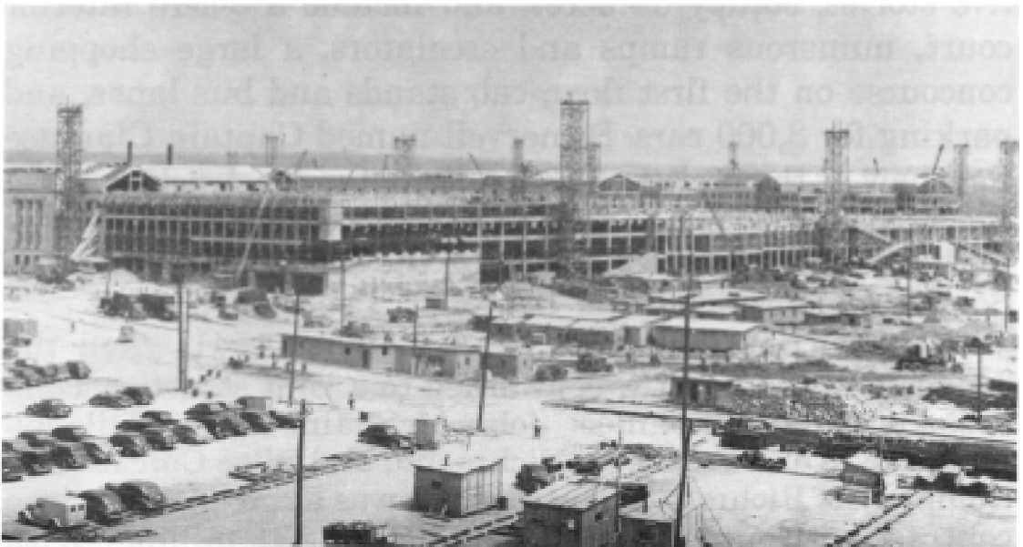
Northwest exposure of the Pentagon construction, 1 July 1942.
