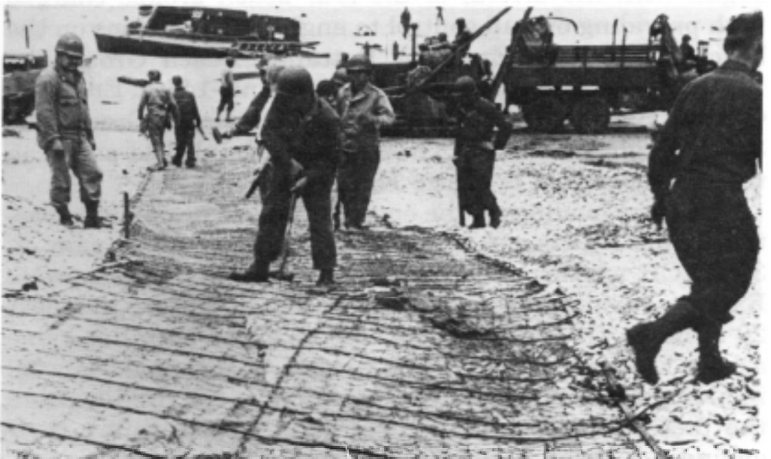
After landing on a beach in France, engineers lay out roads on the soft sands for the heavy vehicles and equipment yet to come ashore, 6 June 1944.
