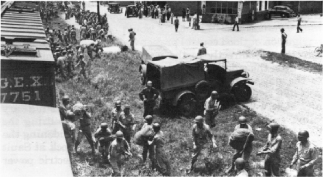
Troops of the 398th Engineer General Service Regiment detrain at Biscoe, Arkansas, to replace the 359th Engineer General Service Regiment fighting the White River flood.
