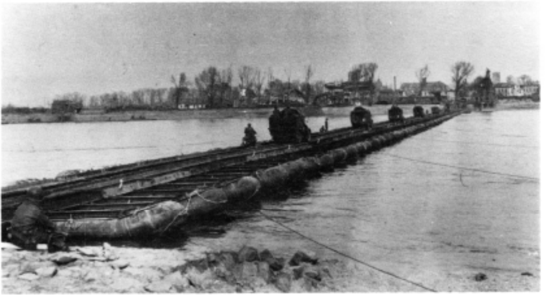
The Ninth Army at Wesel cross the Rhine on a ponton bridge built by the 167th Engineer Combat Battalion, 1117th Engineer Combat Group.
