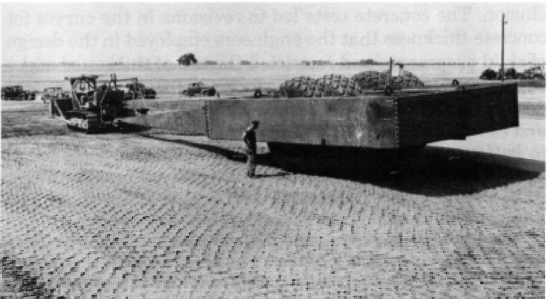
A 120-ton pneumatic roller producing firmly compacted soil.
