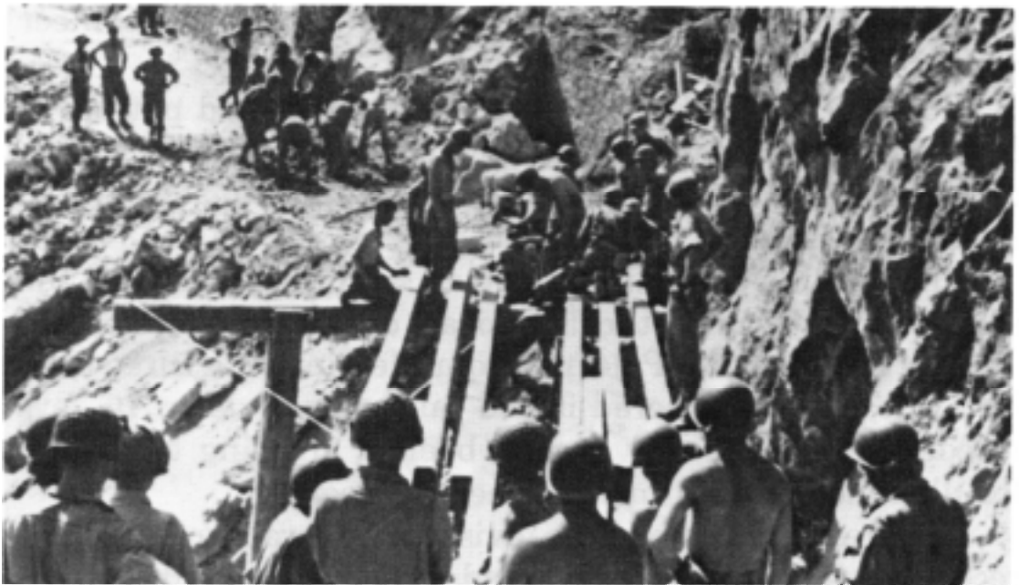
Engineers position stringers on the sky bridge, 13 August 1943.
