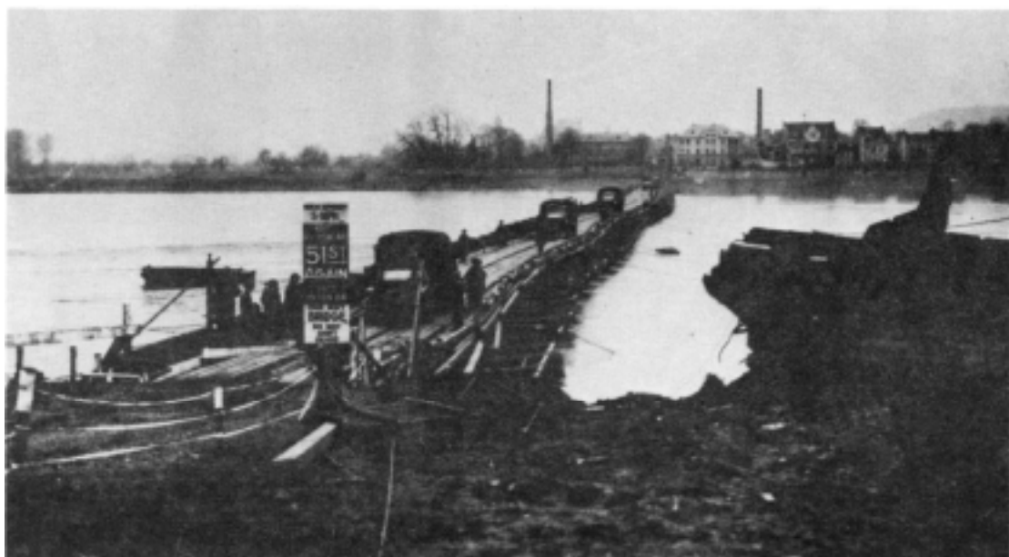
The 51st Engineer Combat Battalion completed the second tactical bridge across the Rhine River at Kripp, Germany, 11 March 1945.
