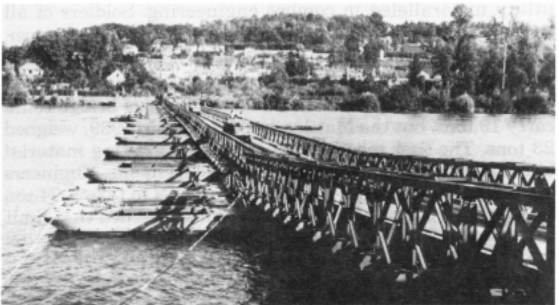
British floating Bailey bridge on Mark VI pontoons. (Engineer School Library)
