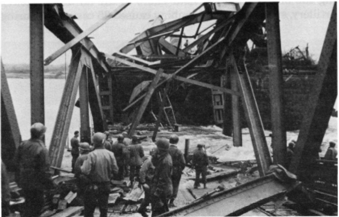
The east end of the collapsed Ludendorff railroad bridge, which spilled several hundred engineers into the Rhine River, 17 March 1945.
