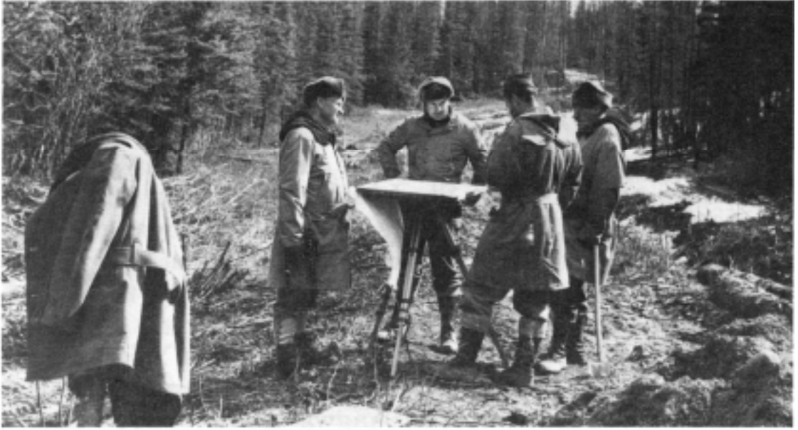
In the northern sector of the Alaska Highway, topographic engineer survey teams work with Public Roads Administration crews to mark locations for the clearing crews.
