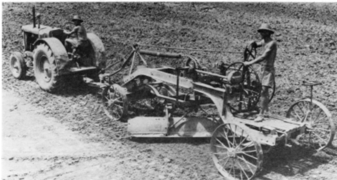
Grading the Mississippi Basin Model site (Waterways Experiment Station)
