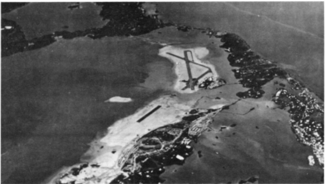
Kindley Field, Castle Harbor, Bermuda, built primarily on dredge fill, April 1942.
