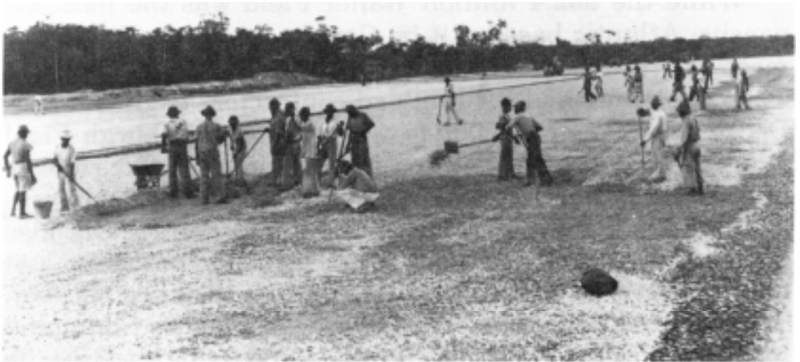
Local workmen construct a runway at Atkinson Field, British Guiana. (U.S. Air Force, National Air and Space Museum, Smithsonian)
